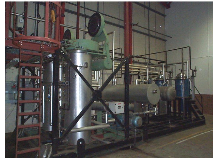
2 x 400 l extraction plant for SCO 2 .
